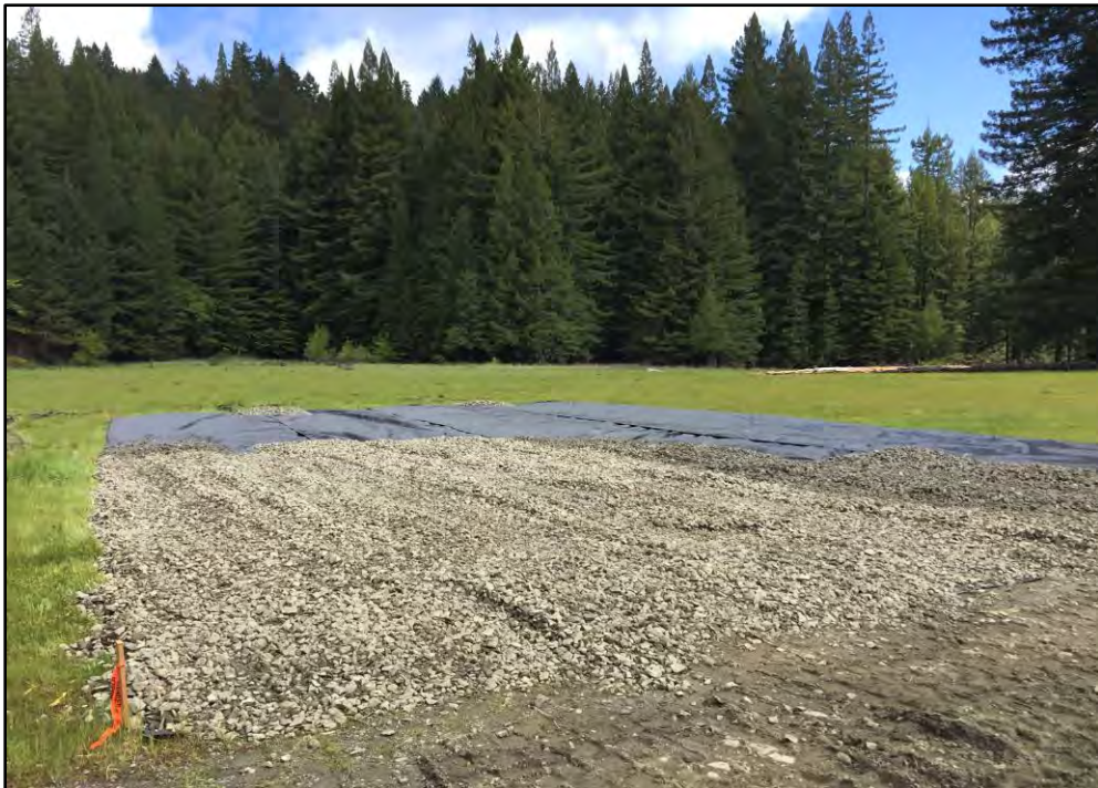
Plastic moisture liner and 2 inch minus rock base is laid for biochar unit.
