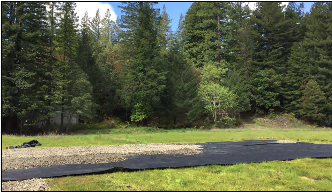
Plastic moisture liner and 2 inch minus rock base is laid for biochar unit.
